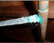
[CR] There is also a section of galvanized pipe being used on the pool house and this is inside the water heater closet and runs to a hose bib. This also has high failure rates and should be replaced. The dielectric coupler in this picture is rusting and failing.
