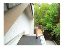
[SC] The vent needs to be extended so that the vent cap or termination is at least 2 feet higher than the elevation of any roof or wall within 8 feet of the vent. The reason is that a wind blowing against the wall could adversely effect the vent and prevent the escape of combustion gas by pushing air down the vent. See section 806.4 UMC-96.
