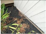
The short wall to in the front is wood framed with a stucco siding and this wall needs the same clearance as any stucco wall.
