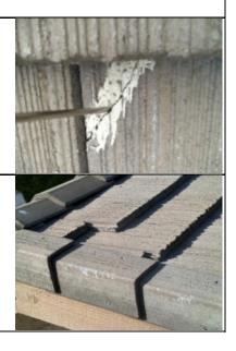
This picture is over the master bath. The tile was not secure along the edge of the wall and moved.
