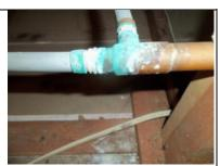
[CR] There is also a section of galvanized pipe being used on the pool house and this is inside the water heater closet and runs to a hose bib. This also has high failure rates and should be replaced.
