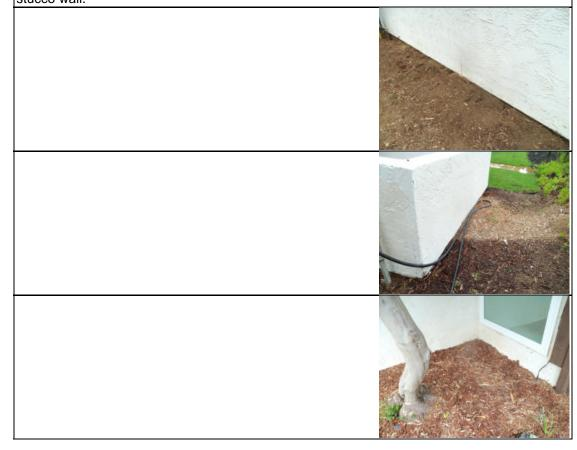
[CR] This picture shows how high the soil level is in relation to the floor level of the pool house. The soil level is too high all the way around and needs to be lowered and the area around this building re-graded. The soil level needs to be a minimum of 6 inches below the slab level. This will be a substantial task.
