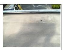
The areas in the picture with the light silt deposits pond water.
