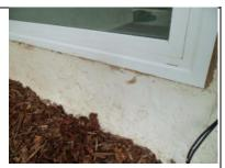
[NOTE] The stucco at the back of the master bathroom extension is crude, uneven and there doesn't appear to be any weep screed and this makes me concerned about the general quality of this addition and makes me suspicious that it wasn't permitted.
