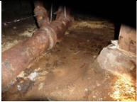
[SC] There is a gas line under this area that is badly rusted and needs further evaluation by a plumbing contractor. This gas line is a couple feet form the toilet so I am not sure how it got rusted. Possibly from leaking below the water heater.
