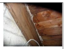
[CR] [CR] Clearly both of the stairs leak and repairs are needed before this can be drywalled. See the deck notes.
