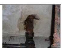
[SC] Repair the damage or holes in the fire resistive wall between the garage and living space.
