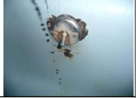
[CR] The tub drained slow. The trap may need to be cleaned or there could be a blockage farther down the drain line. Request that it be clean and free flowing when you move in. Whenever the drain lines are older cast iron, there is always a possibility that this can be an indication of more serious problems which can be expensive to repair. See the note about cast iron in the Plumbing section.
