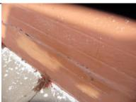
[FE] The portion of the wall closer to the corner has substantial cracks and needs to be considered in an early stage of failing. How long the wall will last is very difficult to predict. It is clearly very weak and the front corner section is badly cracked and has bulged.
